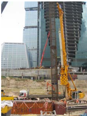
Installation of the reinforcing cage with O-cells
